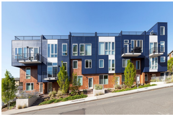
Figure 21. Examples of HardiePanel. This material is not allowed on ground floor façade, but in combination with other building materials (right) can be an effective exterior material above the ground floor.
