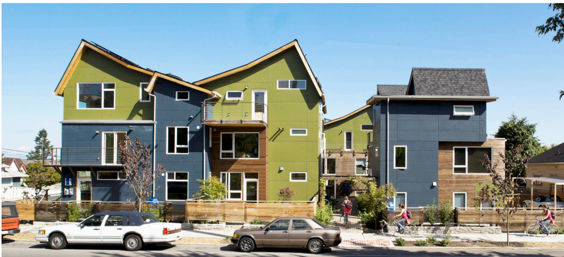
Figure 15. Example of a distinctively designed roofline.
