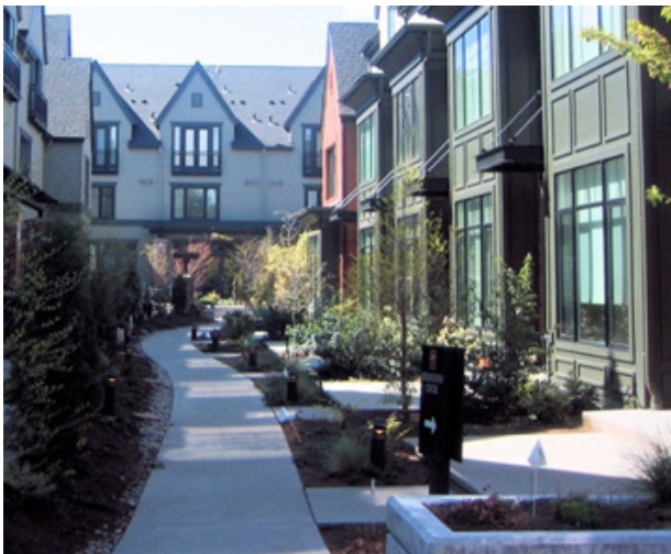
Figure 9. This residential complex incorporates passive surveillance, territorial definition and good visibility and lighting to provide a more secure pathway and open space.
