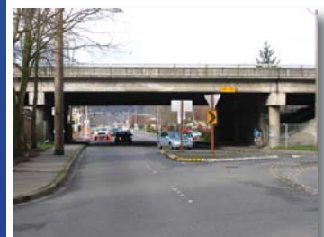
Meeker Street Undercrossing of SR 167
