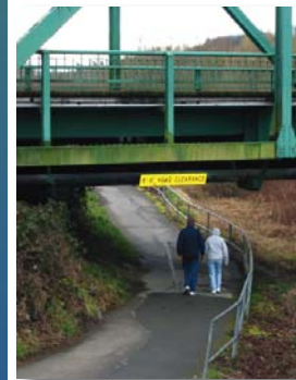
Green River Bridge Connection
