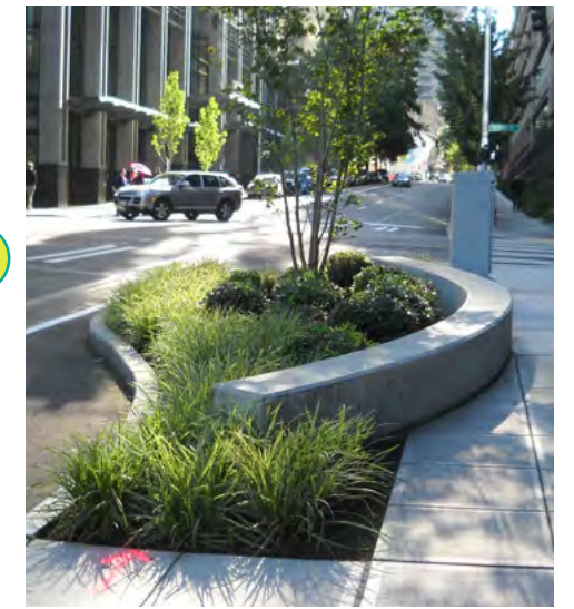
Example of treatments including, roadway lighting, seating, sidewalk treatments and landscaped planters
